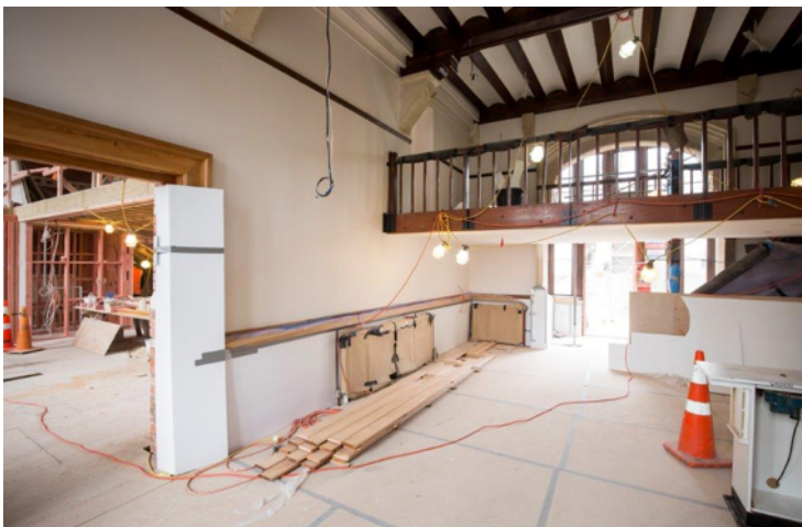
Clock Tower restoration
